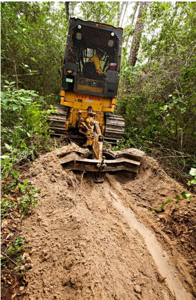
Picture 3. Example of a firebreak installation. Source: SCFC
